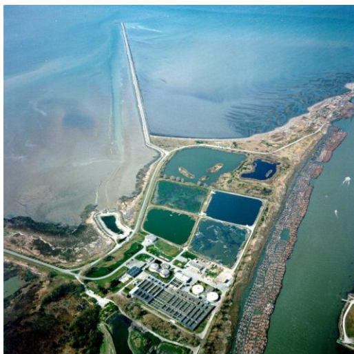
Figure 4: Aerial photo of Iona Island Wastewater Treatment Plant.
