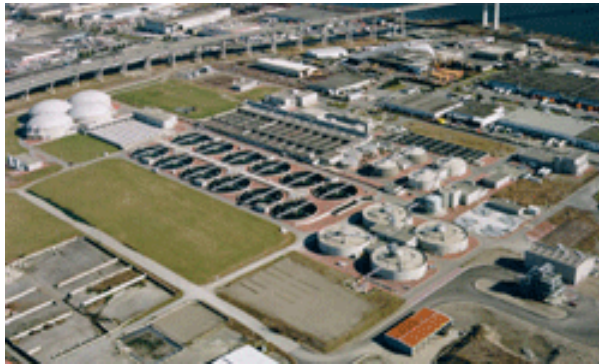
Figure 3: Aerial photo of Annacis Island Wastewater Treatment Plant.
